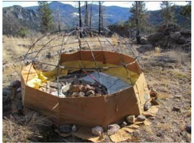
Be thorough in the seal at wall base to stop air and light
